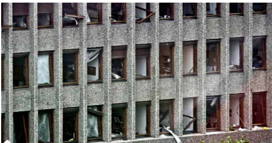
Security film PROFILON® ER1 avoided any life-threatening fragmentation and splintering after the explosion in Oslo.
